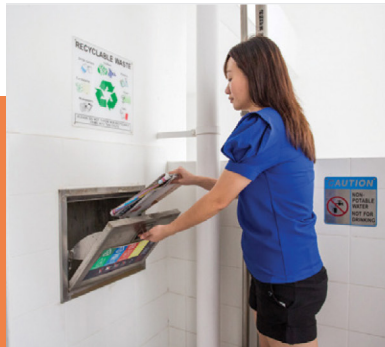
SEPARATE CHUTES FOR RECYCLABLE WASTE
