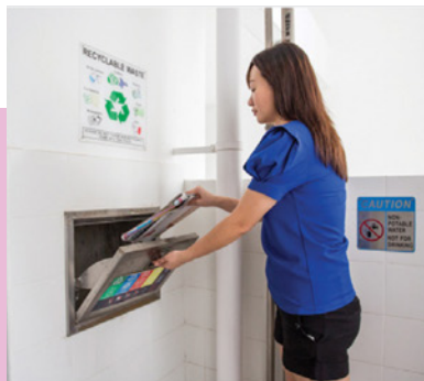
SEPARATE CHUTES FOR RECYCLABLE WASTE
