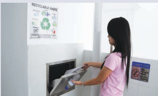
Separate chutes for recyclable waste
